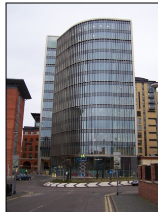
Figure 2: View of completed building
