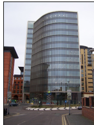
Figure 2: View of completed building
