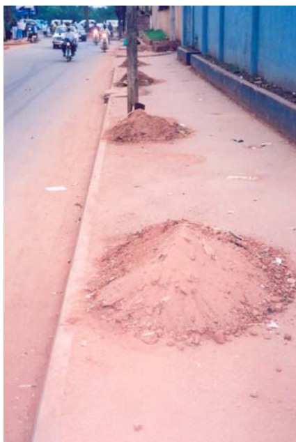
Figure 6. Piles of silt cleared from a drainage channel, Kampala, Uganda (photograph: B Reed)
