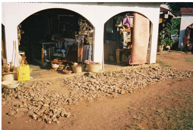
Figure 9. Builders' rubble creates an informal permeable surface, Kampala, Uganda (photograph: B Reed)
