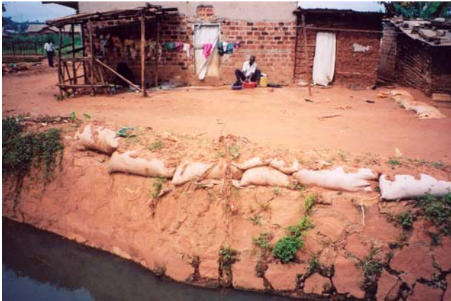
Figure 7. Sandbags protect property from overland flow, Kampala, Uganda (photograph: B Reed)
