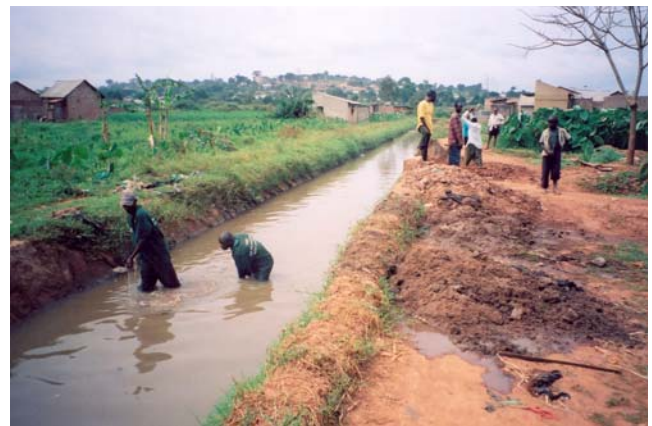
Figure 5. Removing silt from a drainage channel, Kampala, Uganda (photograph: B Reed)
