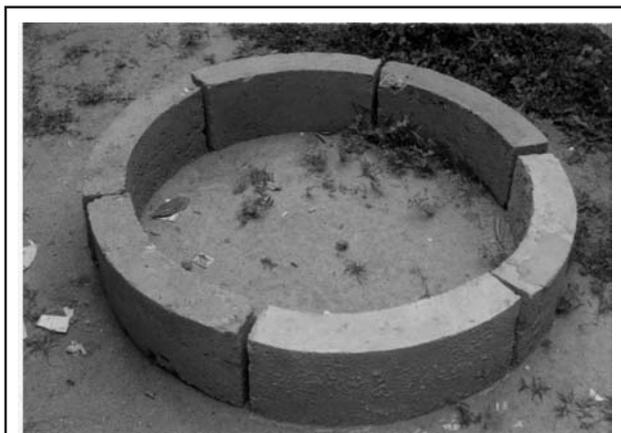
Figure 3. Concrete block option for intake area of a well
