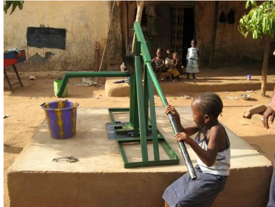
Photograph 1. Improved well with local pump. Well head protection by owner, pump provided by WaterAid
