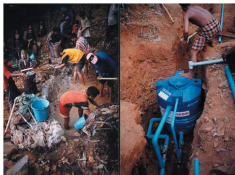
Photograph 2. Building of gabion intake with clay (left) and set up of plastic sedimentation tank (right)
