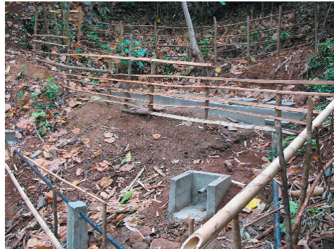
Photograph 1. Concrete intake and its overflow in Namhee Village (6 hrs walk from road access)
