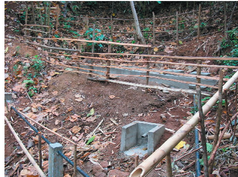
Photograph 1. Concrete intake and its overflow in Namhee Village (6 hrs walk from road access)
