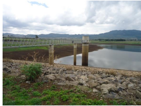
Photograph 2. Dire reservoir area
