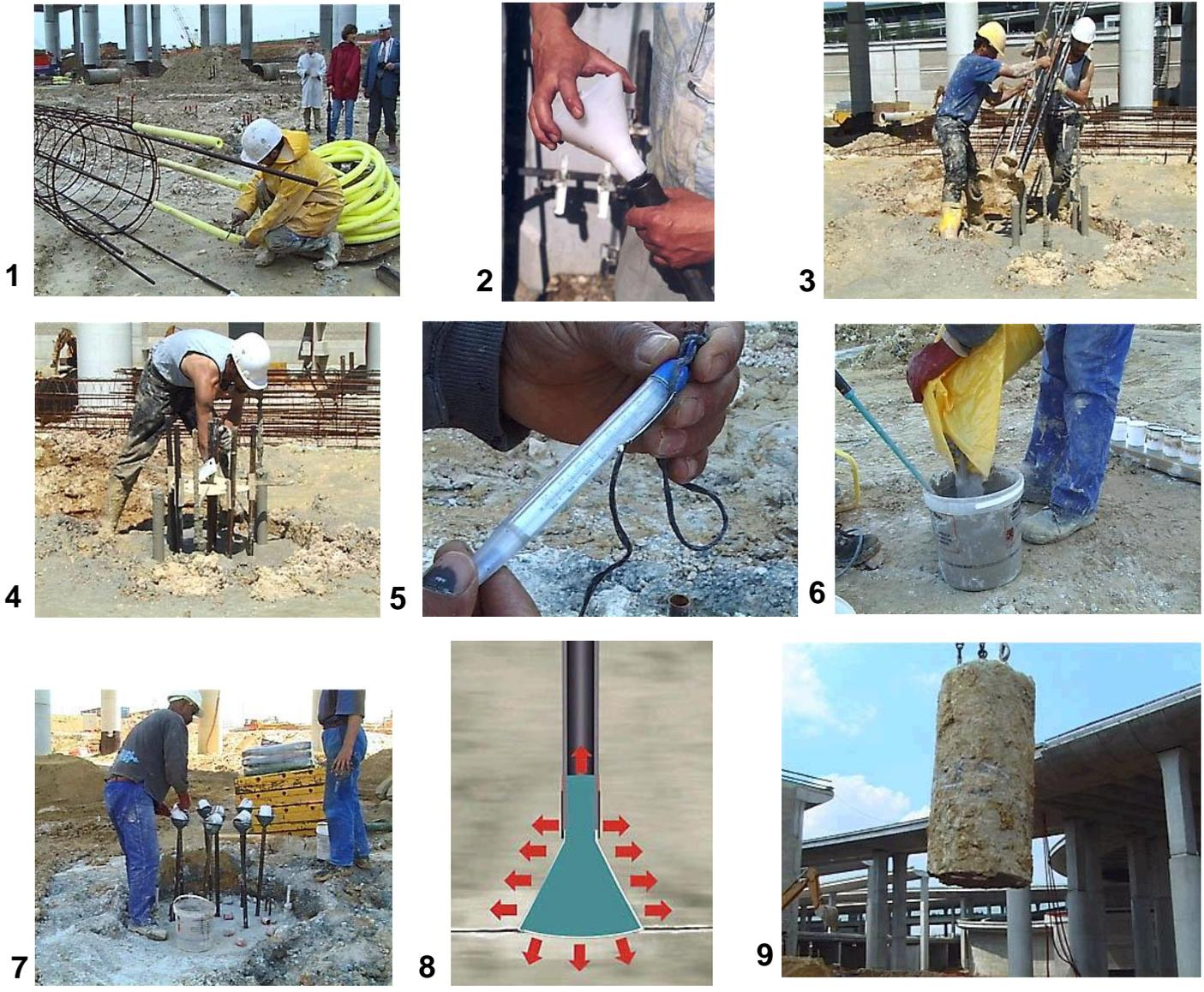
Figure 7 - Recepieux chemical pile breaking method (<http://www.recepieux.com>)
